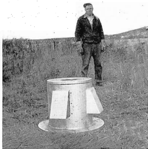
Fig. 9. View of Flange Pedestal Adapter used to mount the UHF Pylon antenna atop the FM Pylon. Wedge-shaped extensions are vent louvers.
