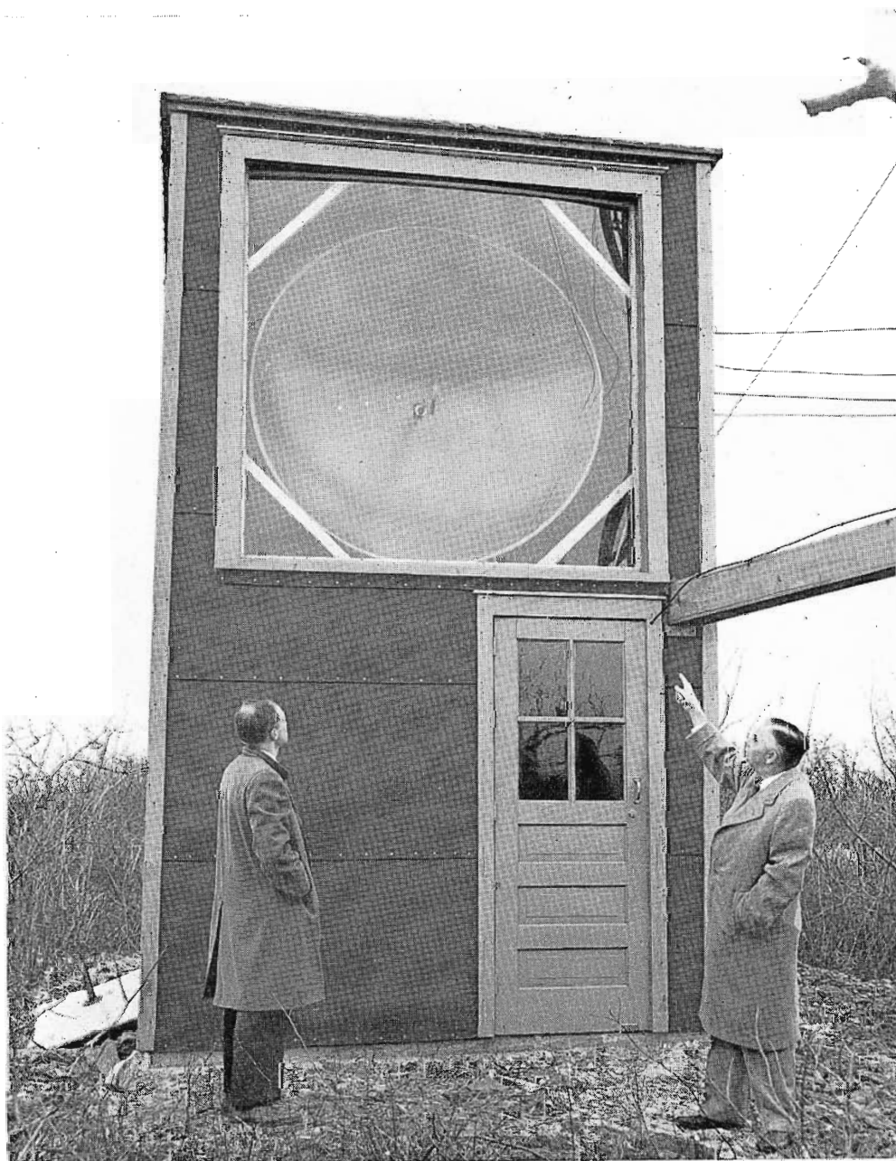
FIG. 7. Relay transmitter housing at Pimple Hill on Effort Mountain. This point is approximately 70 miles from New York and is used as main inter-city relay connection.
